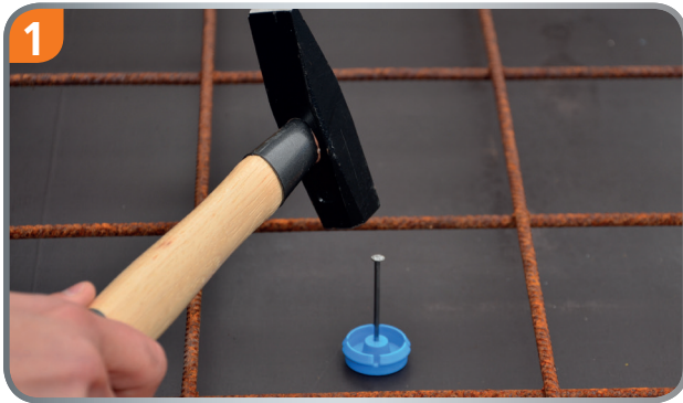
1 Nail the cover on the formwork.
