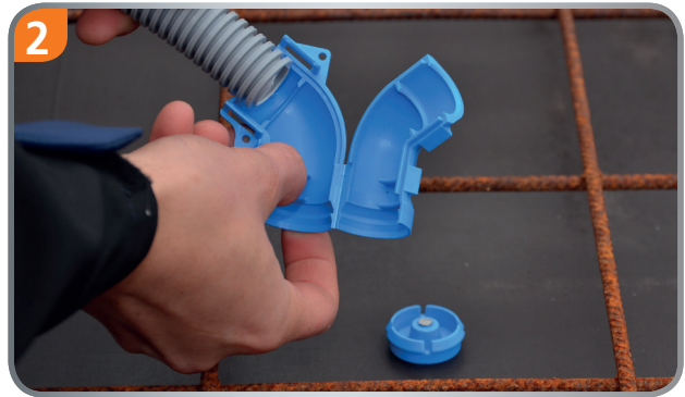
2 Insert the M20 pipe or the M25 pipe.
