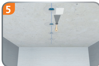
5 You can drill different and individual openings, grout the ceiling.
