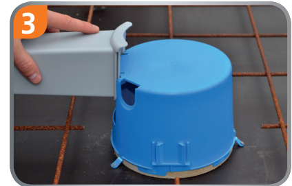
3 Connect the tunnel (SCS-technology).
