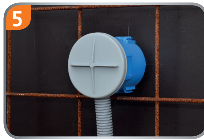
5 Wall installation as electronic box.
