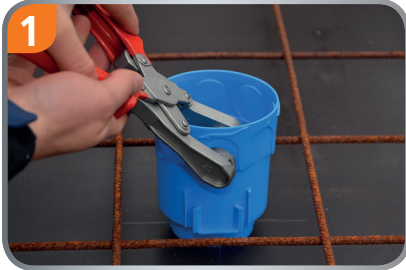
1 Punching a hole for the concrete pipe.
