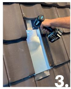
Secure metal tiles to roof battens using sealing screws.
