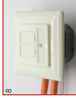
8 Aussembling Adapterplatte und Zentralplatte befestigen / Fasten cover plate adapter plate, and mounting plate
