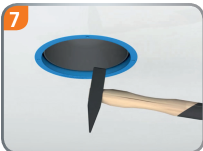
Open the bottom of the ventilation sleeve with a hammer.
