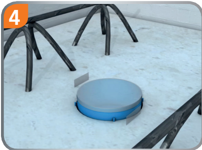
Remove the protection cover from the ventilation sleeve.
