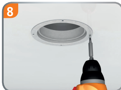
Install the ventilation output connector.
