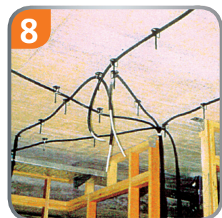
8 Also to fix more cables in a drop ceiling
