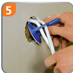
5 Drag out the cable holder.
