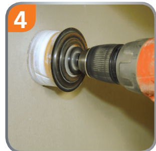
4 Drill a 68mm hole without measure.
