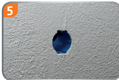
5 Now you can fill the thermal insulation and plaster.
