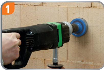
1 Mark the first box and drill a \varnothing 82 mm hole.
