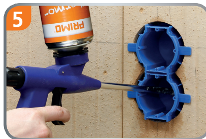
5 Lathering the box, the side clips set the plaster thickness.
