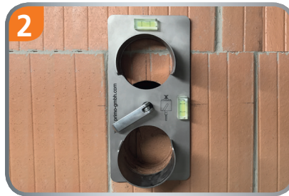
2 Insert and adjust the drilling template and drill another holes.
