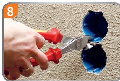
8 Remove the SCS connection after plastering.
