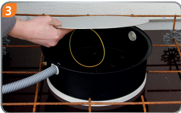
3 Insert the concrete pipes and fix the cover on the light-box with the included accessories.
